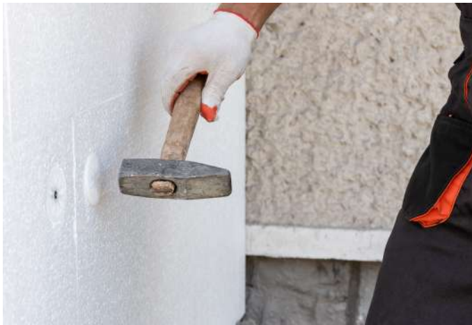
Example of a properly installed anchor
