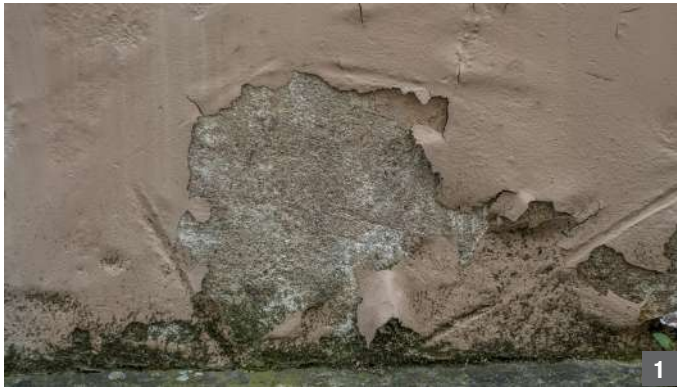
Moisture in the substrate
