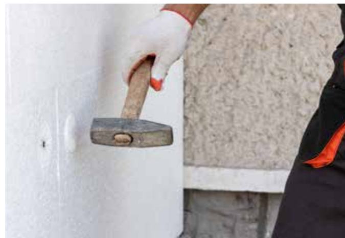
Example of a properly installed anchor
